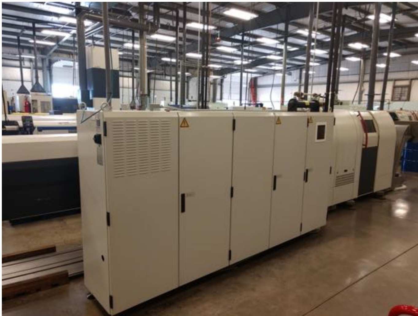
Power supply for TNL26 S/N 160
